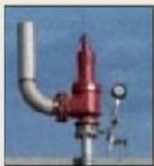
Photo of a pressure relief valve
