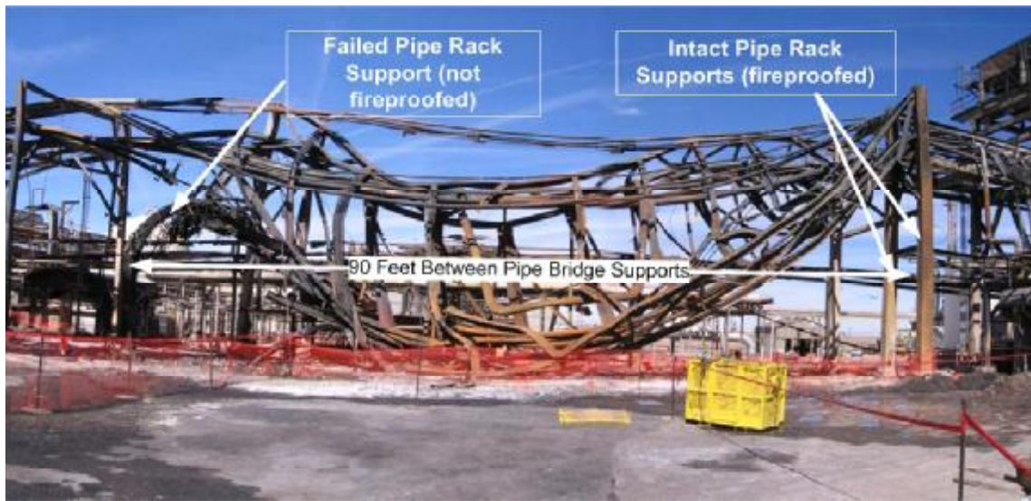
Figure 9. Pipe bridge support fireproofing
