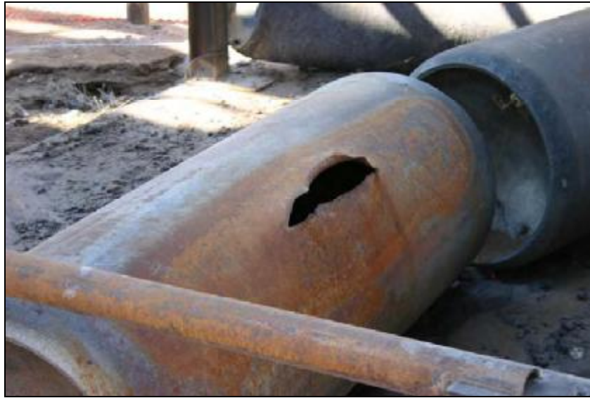
Figure 13. Ruptured one-ton chlorine container
