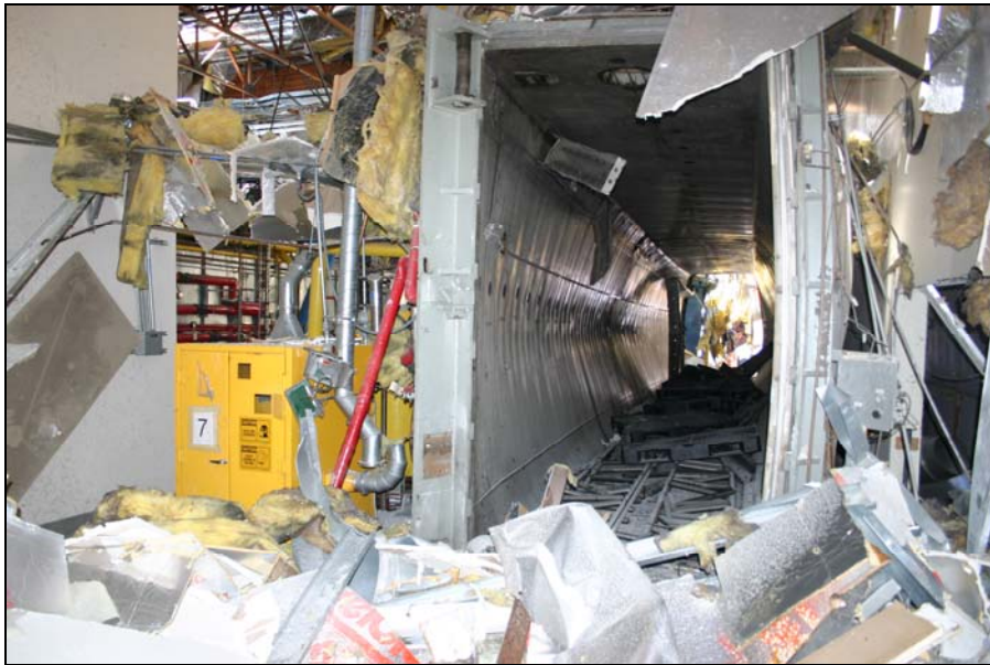
Figure 13 Damage to Sterilization Chamber 7
