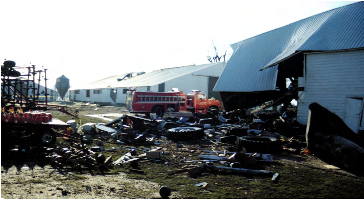
Figure 13. Southeastern View of Damage to Workshop Caused by Impact of Large Tank Fragment
