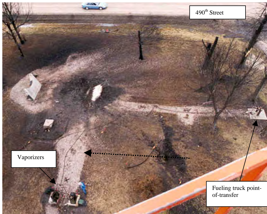
Figure 7. Aerial View of Tank Area
